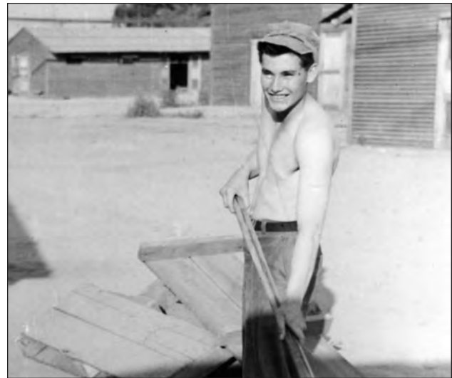
Herb building a sidewalk.
