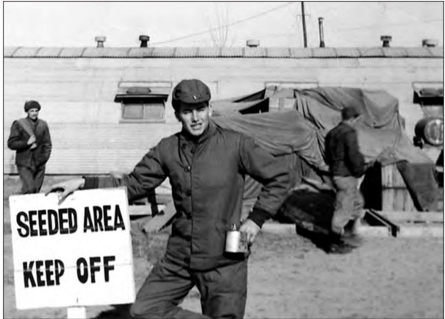
Herb, holding his canteen, takes a break from building a gravel sidewalk beside the Quonset hut in background.
