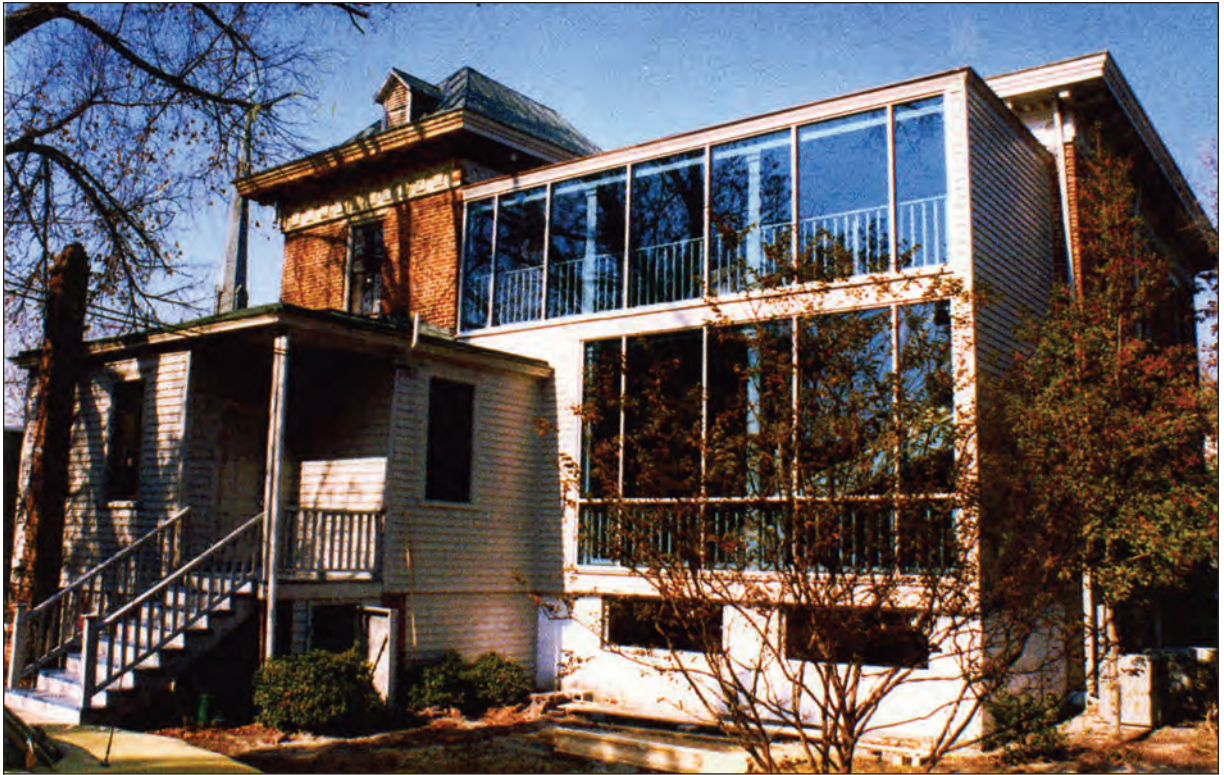
Rear of the BMS Market Street office. Built in 1856 across from Bellamy Mansion, Herb and his colleagues revised the rear elevation to increase floor space.
